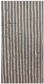
Detail of a wall, Vindebrogade
